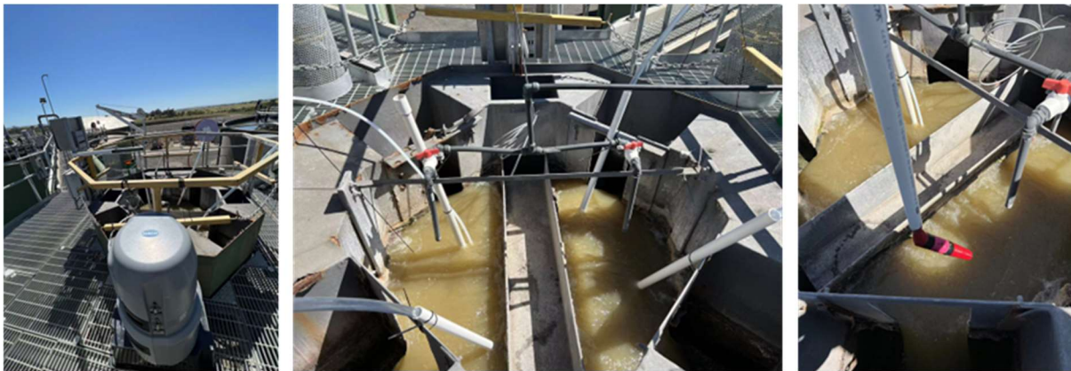
Figure 2. MAD-AS validation set up in the wastewater treatment plant. Hach SD900 autosampler (grey machine) sitting in front of the lagoon (left picture); MAD-AS sitting in the lagoon (tubing come out from the white PVC pipes), the tubing is connected with the MAD-AS and fixed on the rail to avoid it flowing away, PVC pipe is used for fixing the tubing at the right place (middle picture); MAD-AS connecting to the tubing which is covered by a PVC pipe (right picture).
